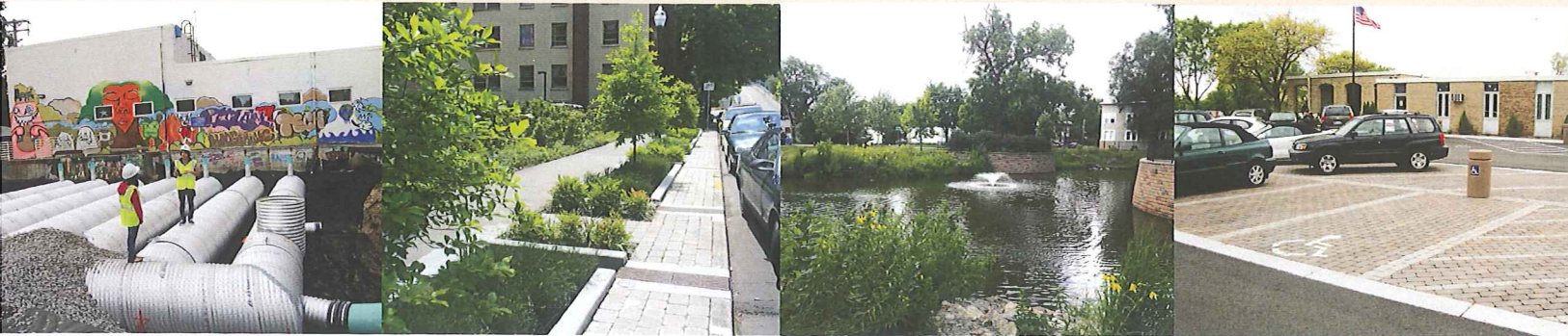
From left to right: Underground filtration and storage, El Colegio High School, Minneapolis (Credit: MCWD), Green street planters (Credit: U.S. Environmental Protection Agency), Wet detention pond, Minneapolis (Credit: City of Minneapolis), Permeable pavers, St. Mary's Greek Orthodox Church, Minneapolis (Credit: Solution Blue)
